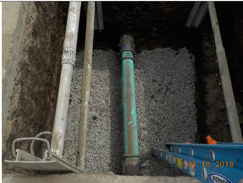
TYPICAL SANITARY SEWER POINT REPAIR – PVC PIPE
